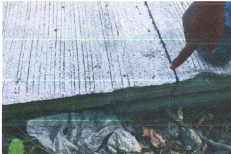
Transverse Cracks
