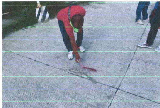
Transverse Cracks
