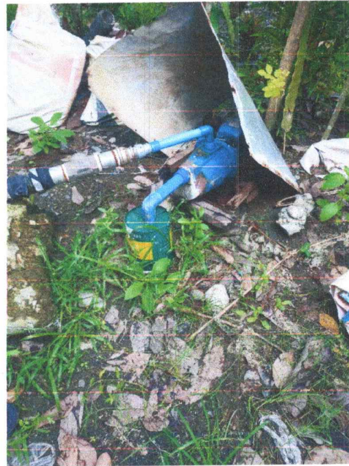
Non-functional Submersible Water Pump
