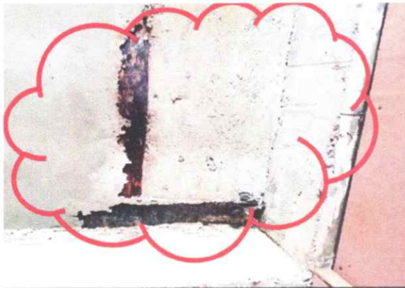
Protruding rebars and unfinished surface
