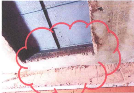
Protruding rebars and unfinished surface
