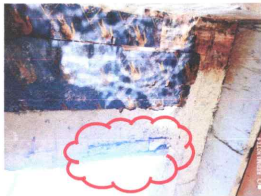
Not removed Frameworks
