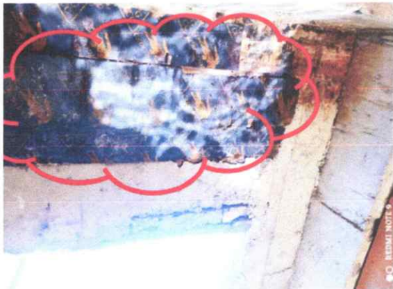
Protruding rebars and unfinished surface
