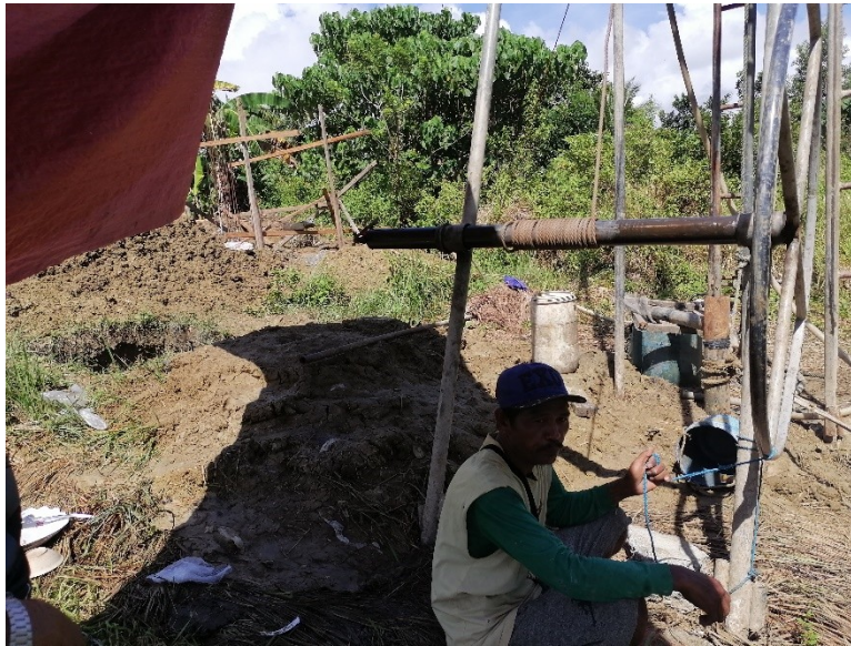
Ongoing/Incomplete drilling works
