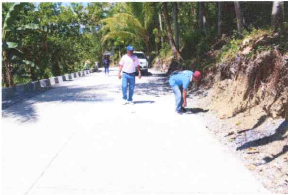
Insufficient backfilling of aggregates on the road shoulder
