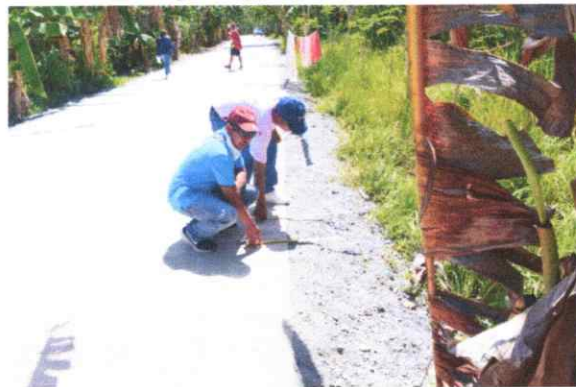
Insufficient backfilling of aggregates on the road shoulder
