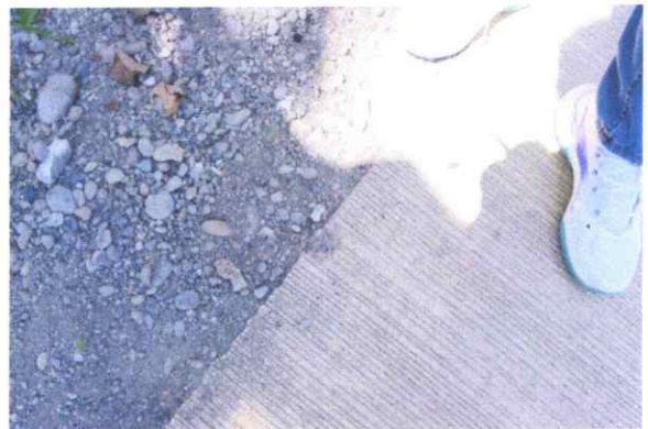
Insufficient backfilling of aggregates on the road shoulder
