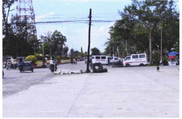
Presence of Electric and Telecommunication post in the Road Right of Way
