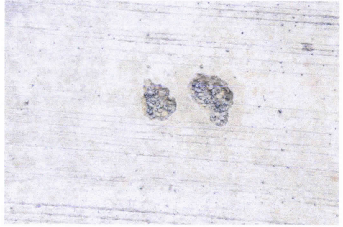
PCCP blocks with pockmarks
