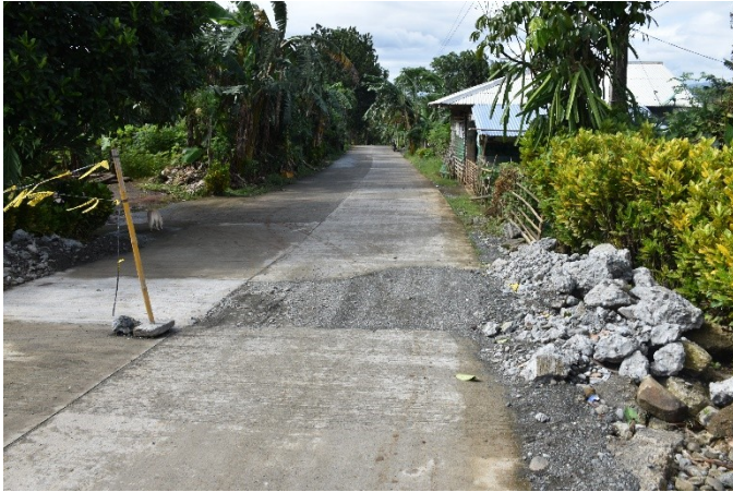
PCCP blocks with on-going Remove and Replace Work
