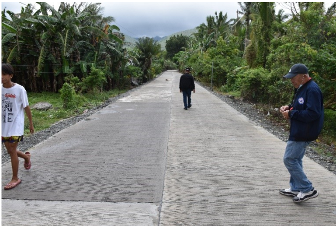
PCCP blocks with application of concrete mixture subject for observation until the next PMC Monitoring Activities.
