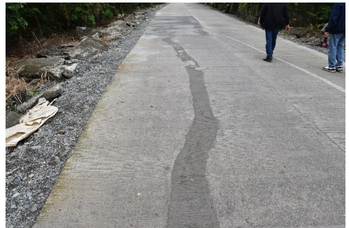
PCCP blocks with application of concrete mixture subject for observation until the next PMC Monitoring Activities.
