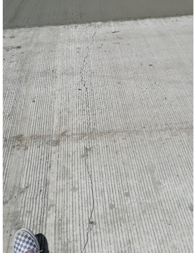
Transverse crackings
