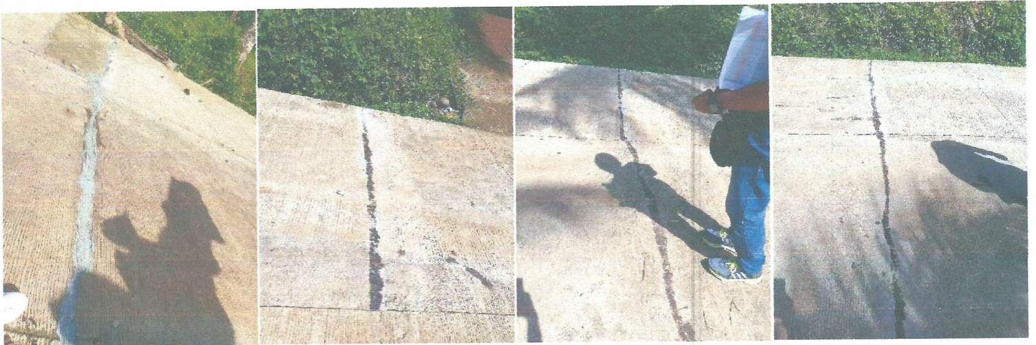
Application of Asphalt Filler and Concrete Epoxy
