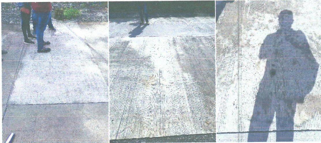
Remove and Replace Works
