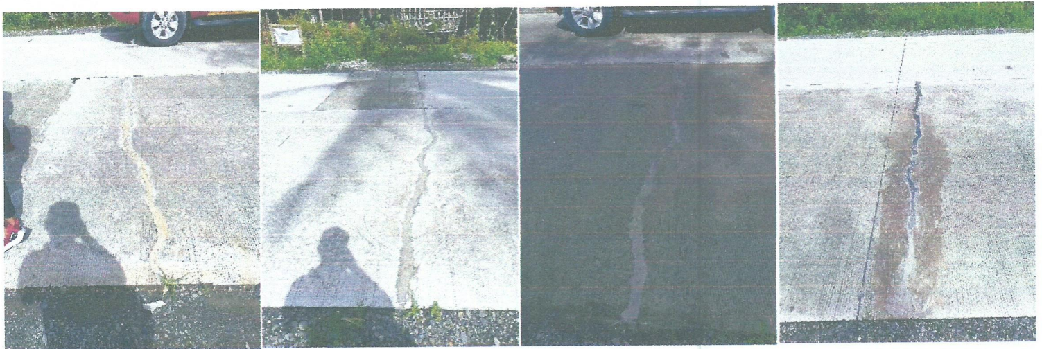
Application of Asphalt Filler and Concrete Epoxy
