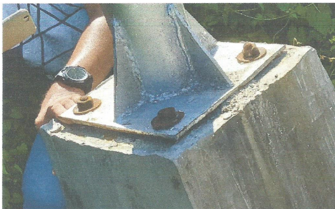
Some base plates are not fitted right with its concrete base/pedestal
