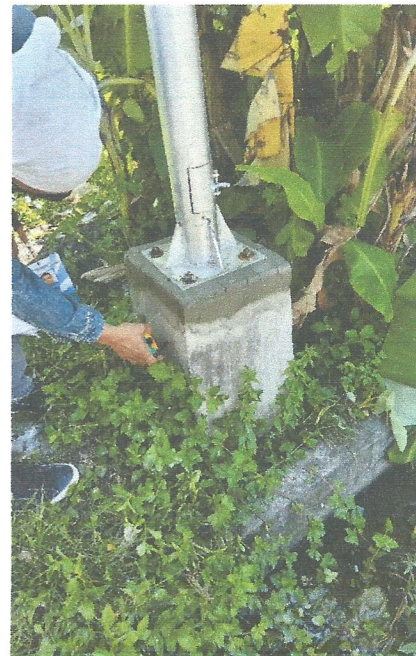
Some base plates are not fitted right with its concrete base/pedestal
