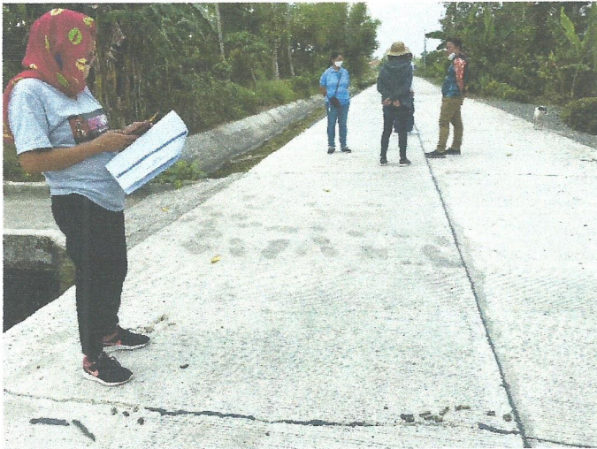
Poor application of asphalt filler
