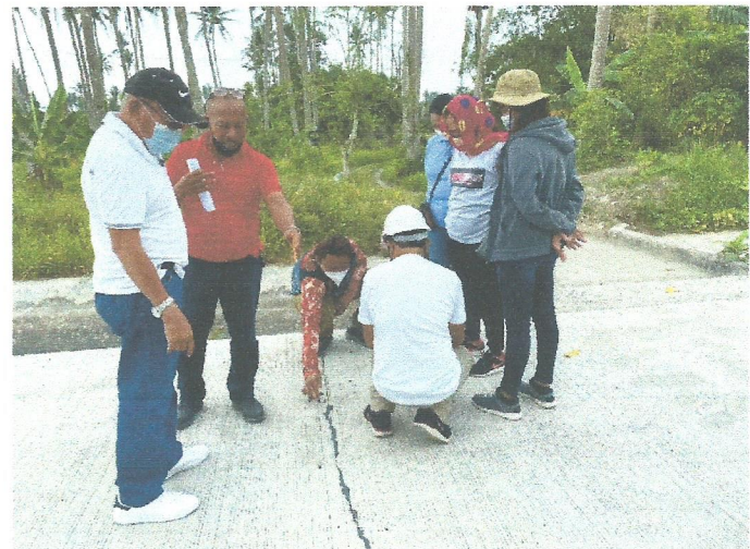
Poor application of asphalt filler
